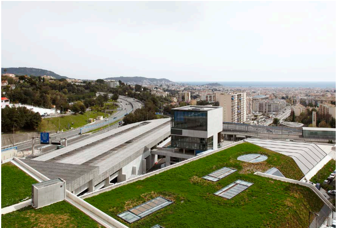
Tramway Terminal, 2007 Nice, France
