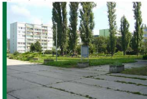
Experimental housing estate Invalidovna, 1960-65 Jiří Novotný, Stanislav Horák, František Šmolík Approximately 1260 apartments for 4200 people
