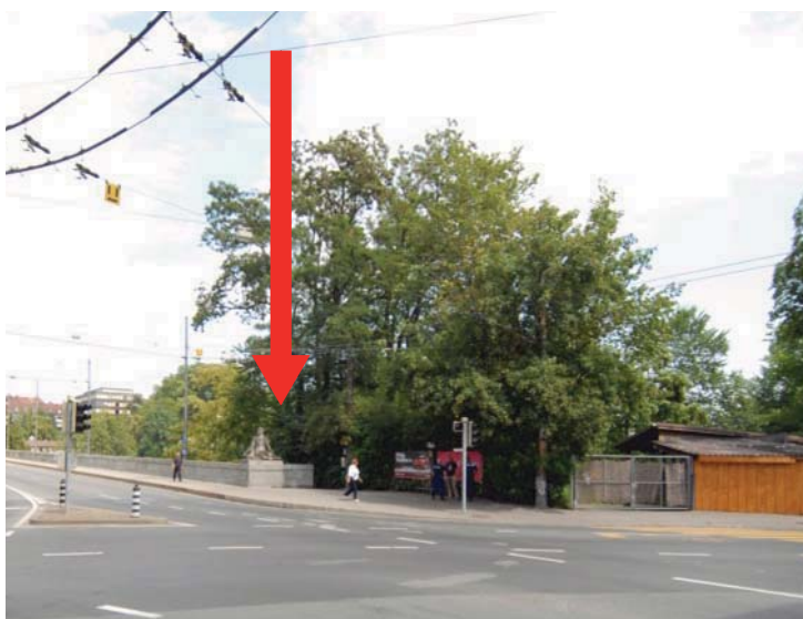
Fig 26 The stair to the river hidden behind the abutment of Lorraine Brücke
