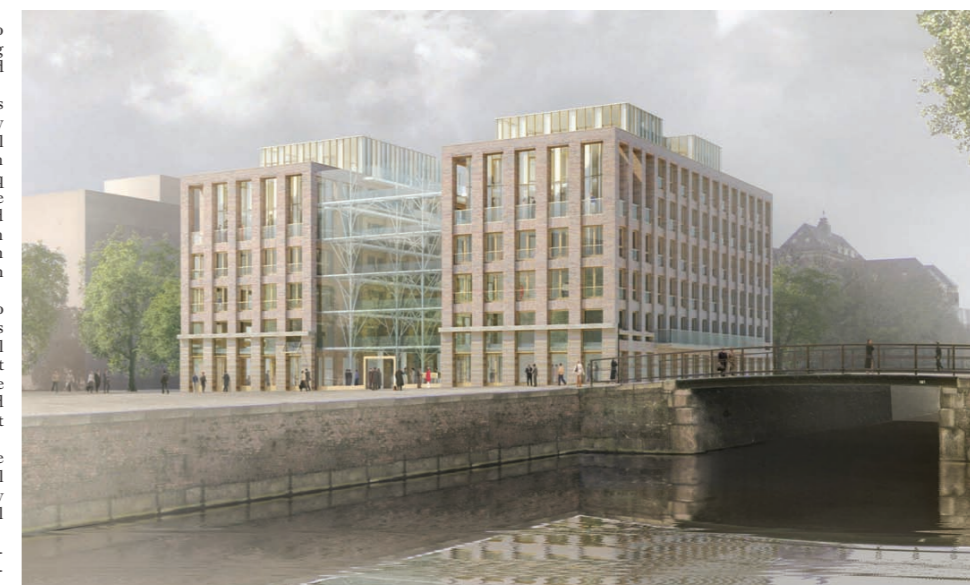
Fretton's building, near Amsterdam's Vondel Park, is comprised of two blocks divided in the middle by a central courtyard.
