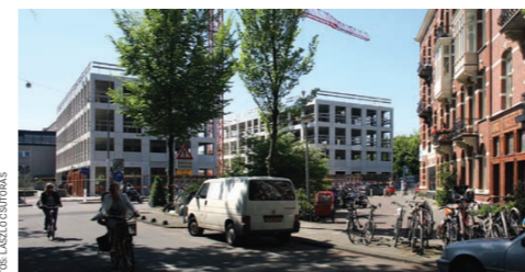
Fretton's blocks under construction.
