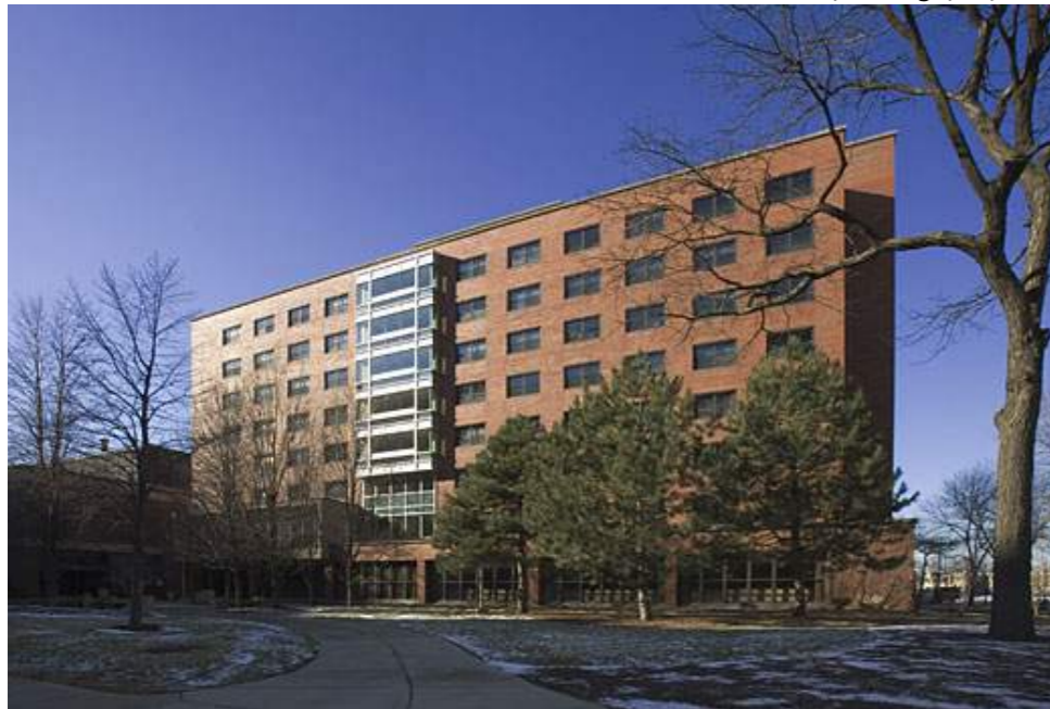
West Residence Halls University of Illinois at Chicago West Polk street, Chicago, IL, USA
