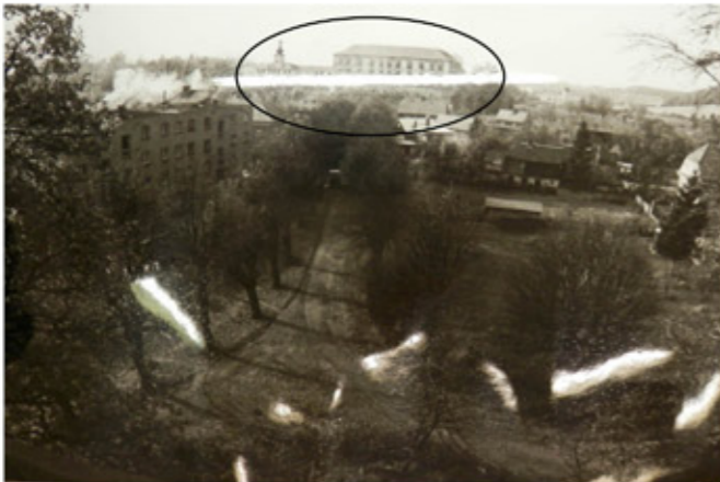
View from the upper window of the church
