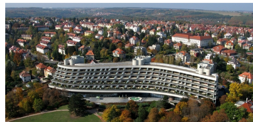
Hotel Praha, 1981, Praha, demolice 2014
