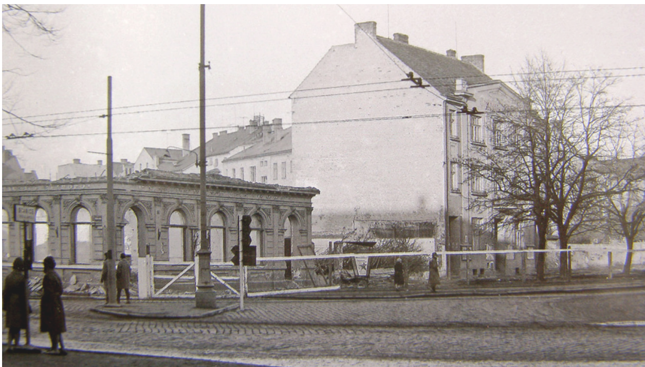
Demolice restaurace Metropol
