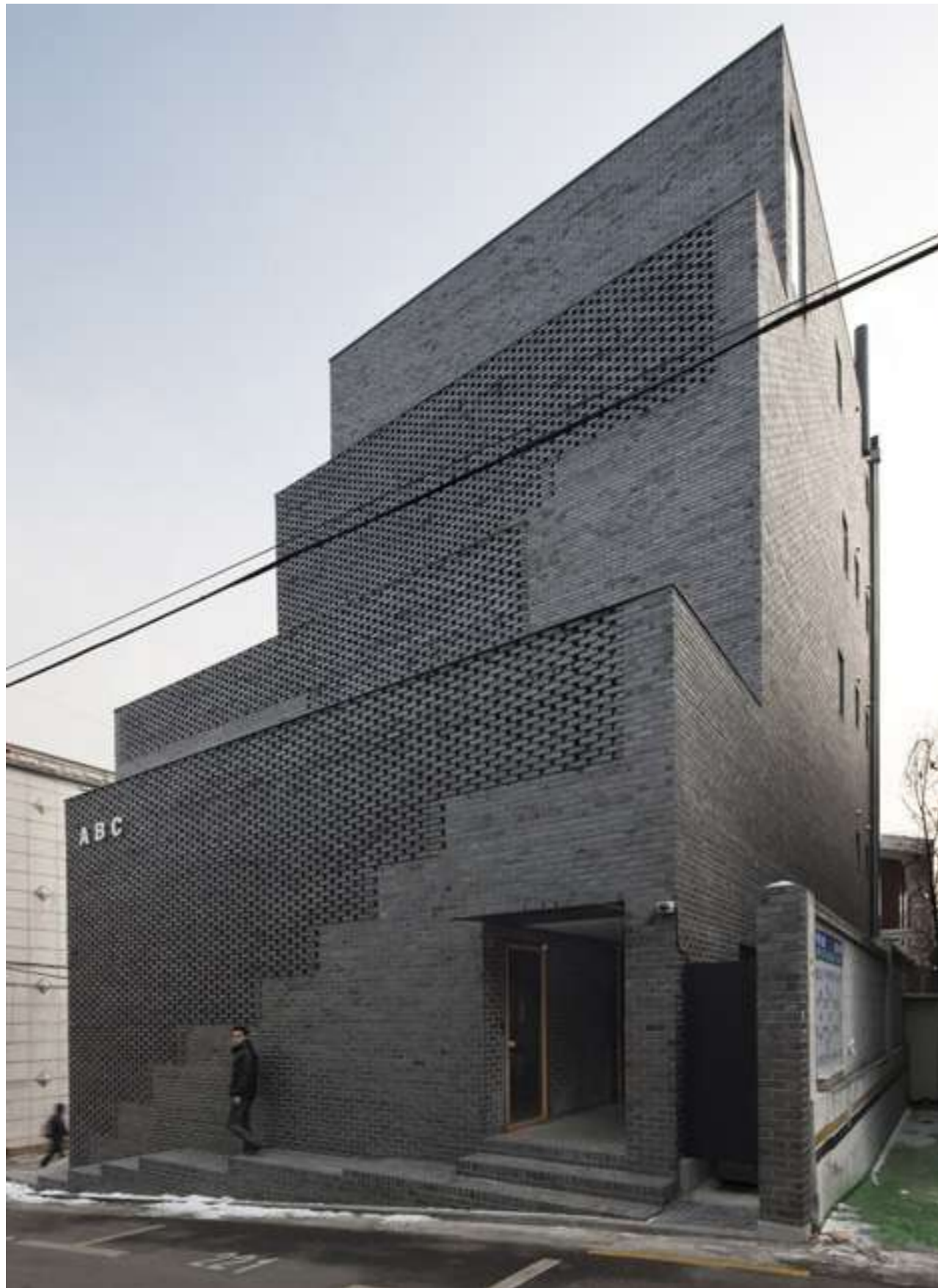
ABC Building / Wise Architecture
