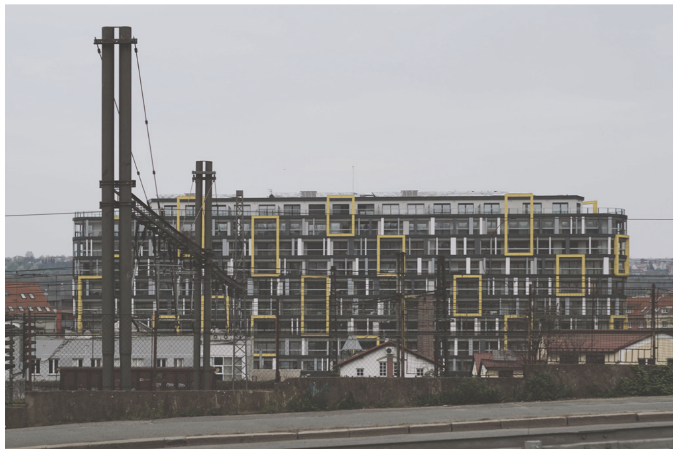
nová budova Harfa Design Residence
