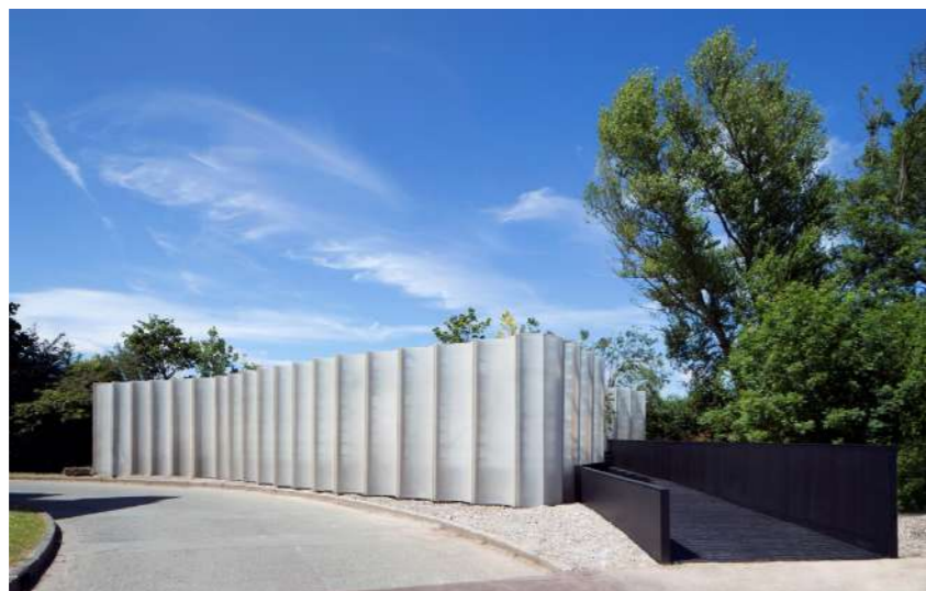
Obr.22 vstup_ maggie's centre merseyside
