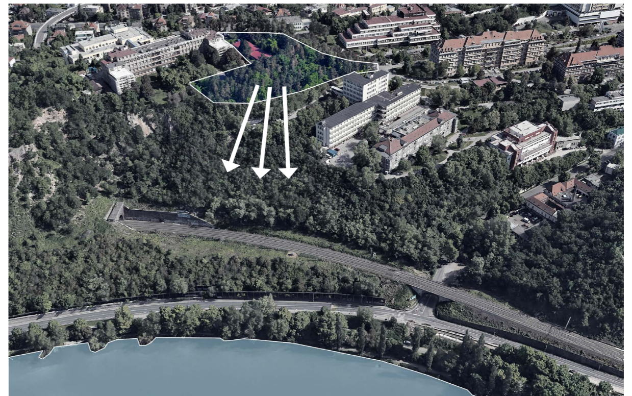
Aerial view A; the project area is located on a hilltop in Bulovka
