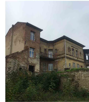
from courtyard to west
