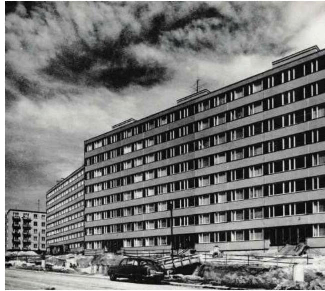
“T08B” in Havířov, experimental bending of the building xvi
