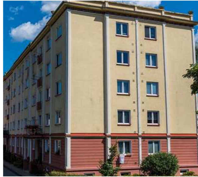
The current appearance of the segmented facade of the “G40” system xxi
