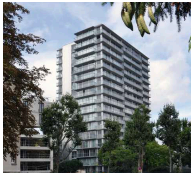
Roof structures and loggia extensions xvi
