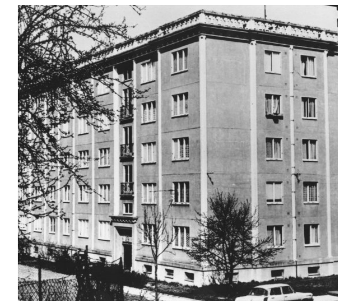
Sample of the profiled main cornice of the house “G55” in Zlín*
