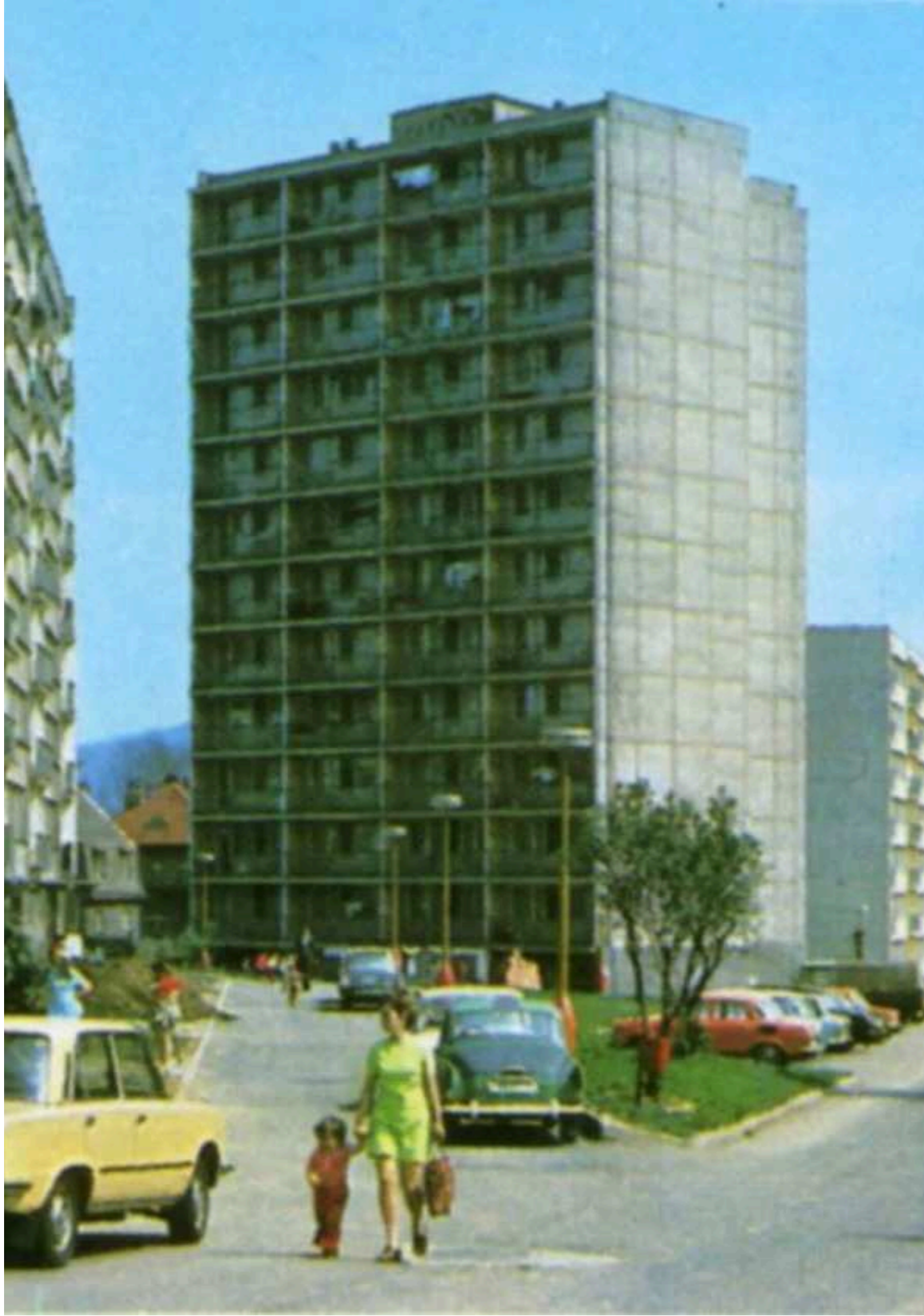
T06B panel houses in the Františkov housing estate in Liberec during the 1970s lv
