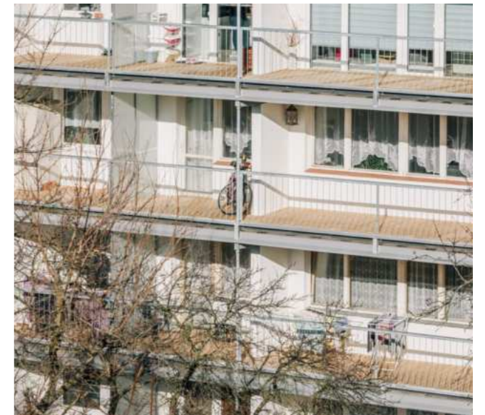
Details of windows and openings to the loggias xl
