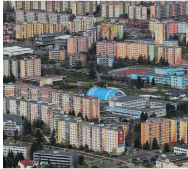
Current state of „T06B-PL“ façades, Plzeň xxix
