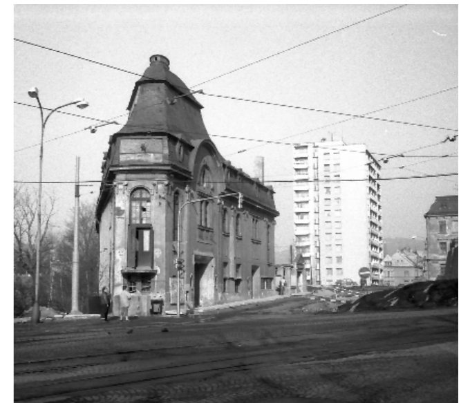
Former Sofia Cinema close to one of the first high rise panel building xii
