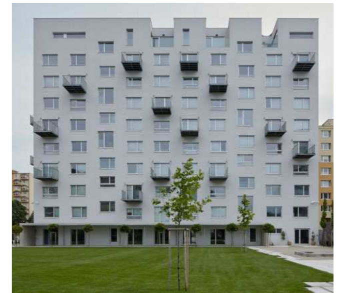
Roof extension and enlarged balconies xvii
