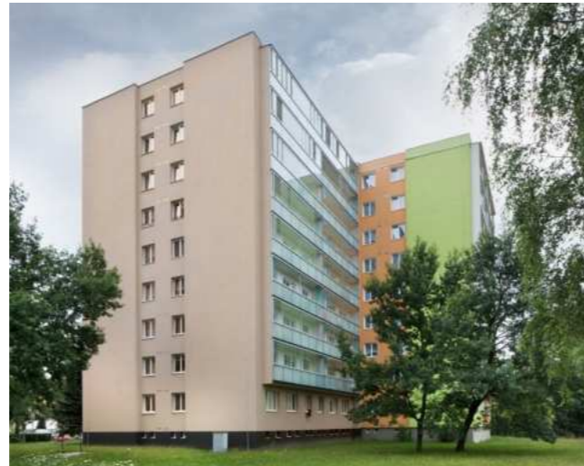
Thermal insulation with new plaster and loggias xxxvii
