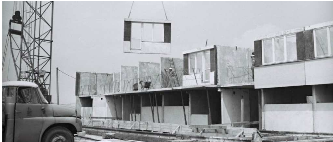
Installation of the peripheral part of the system „T06B OS 70“ 16
