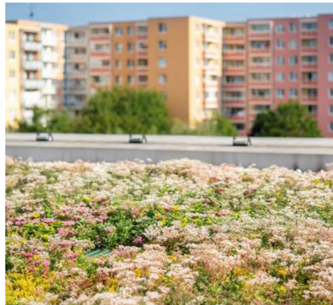
Extensive greenery on a panel house in Brno-Bohnice xiii
