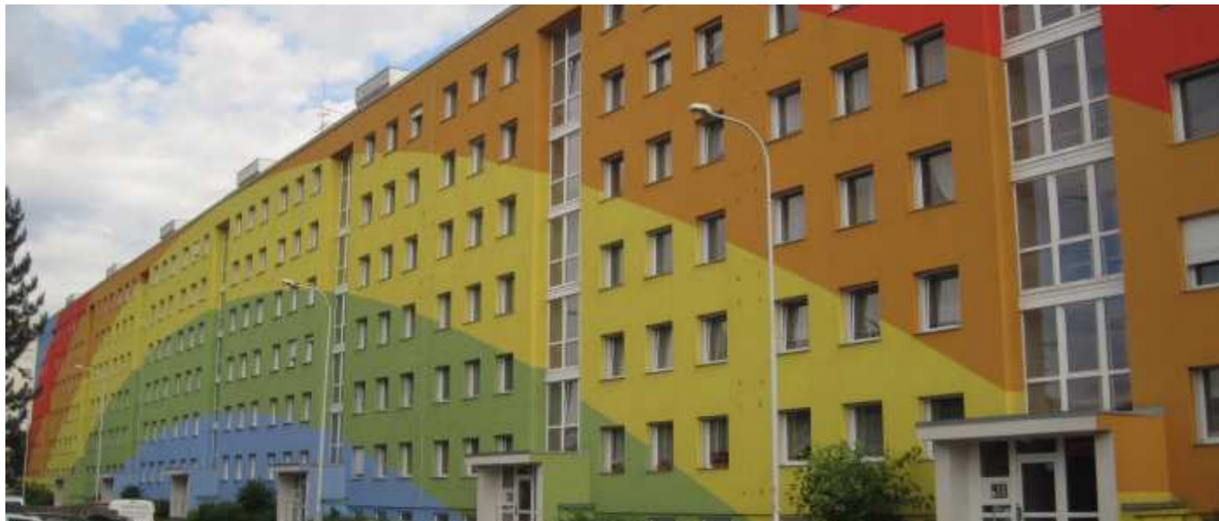
Rainbow facade of an insulated panel house in Prague xiv
