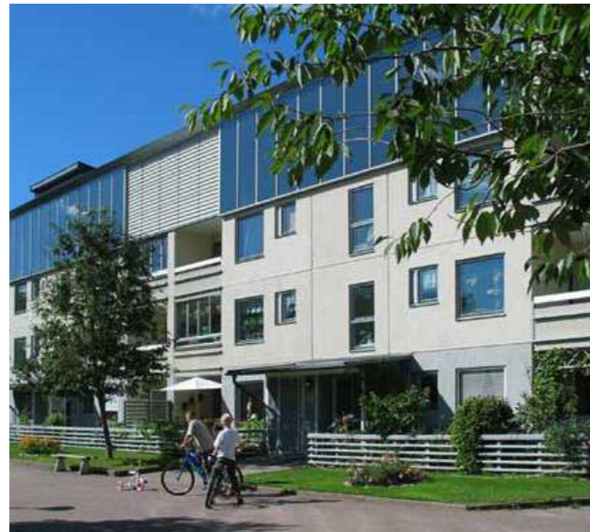
Facade photovoltaic panels vlix
