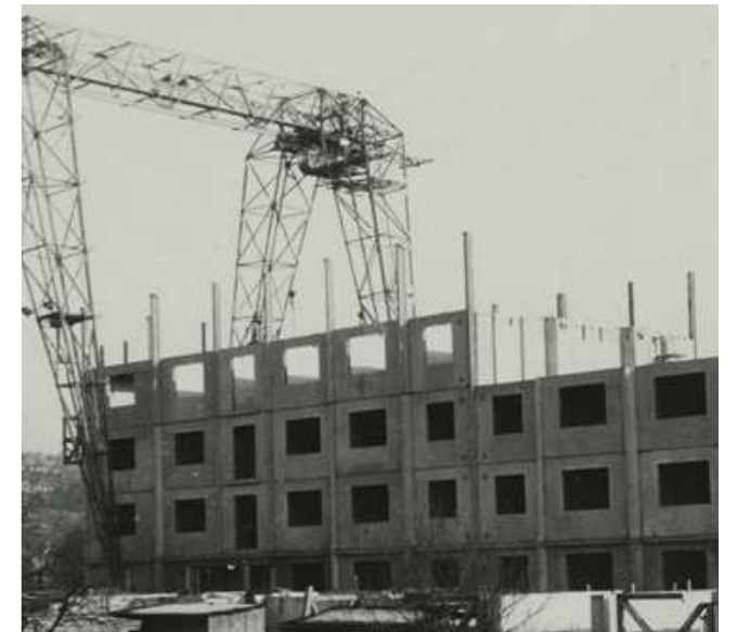
Construction of a panel house type “G40”, Zlín 1953 18
