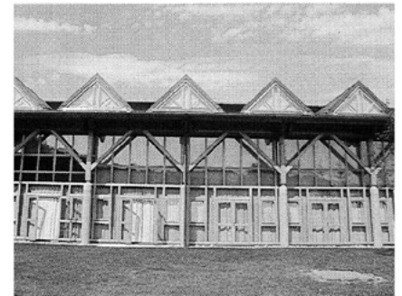
Continuous triangulated structure in the wall
