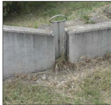
Photo 10. Kronsberg. Swales are located along a sloping terrain and concrete weirs are implemented downhill to avoid too large runoff flow rates.
