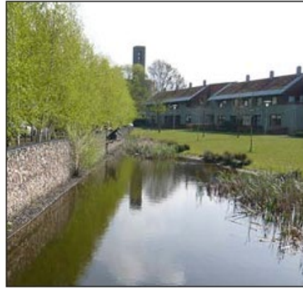
Photo 7. Monnikenhuizen. Infiltration pond for stormwater runoff with low water level after a longer dry period.
