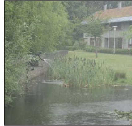
Photo 8. Monnikenhuizen. Infiltration pond for stormwater runoff during a rain event, which results in a higher water level and the sculpture spewing water.
